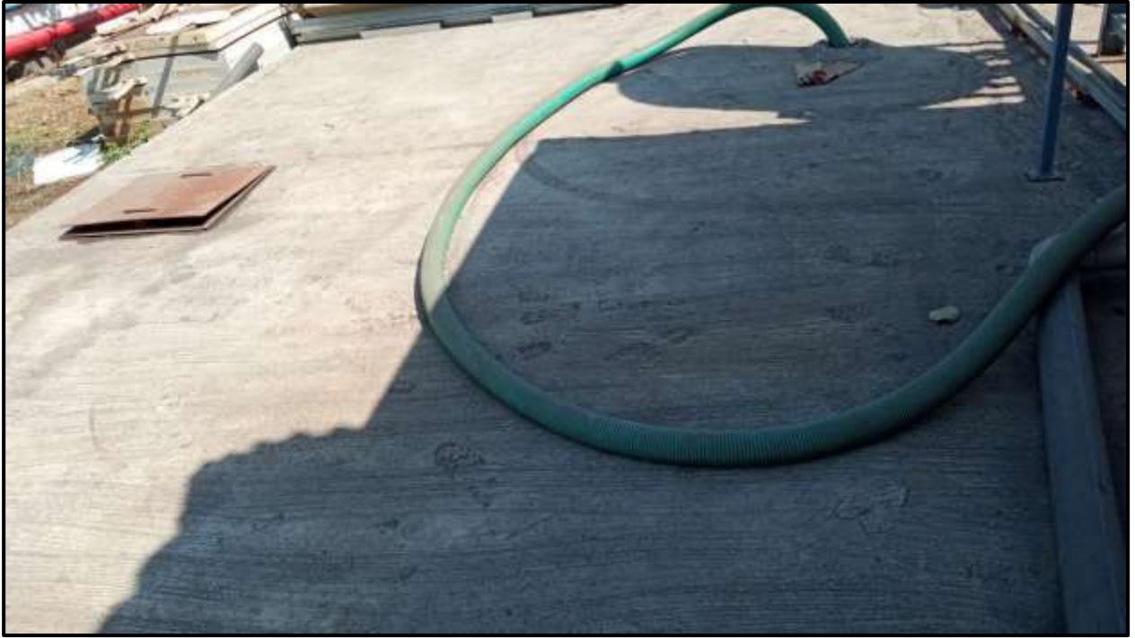
Rain water harvesting Tank
